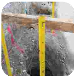
Using a string line, set out post holes to suit sleeper length. Holes are dug at 450mm diameter for all walls up to 1.6m. Hole depth is equal to wall height plus 200mm. Add 600mm if fence being attached
